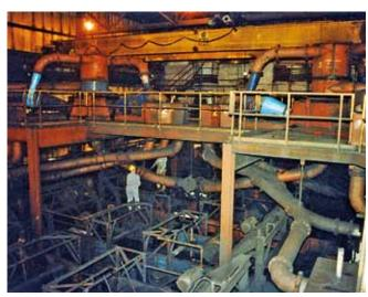
Hydraulic conveying pipes integrated in a coal preparation plant in North America. The pipes have been lined with ABRESIST. In this case they reach service cycles of more than 20 years.
